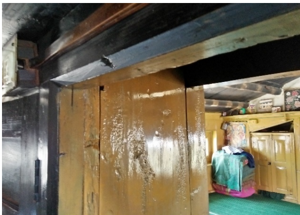
Fig. 18: Wooden Lintel over the Door
