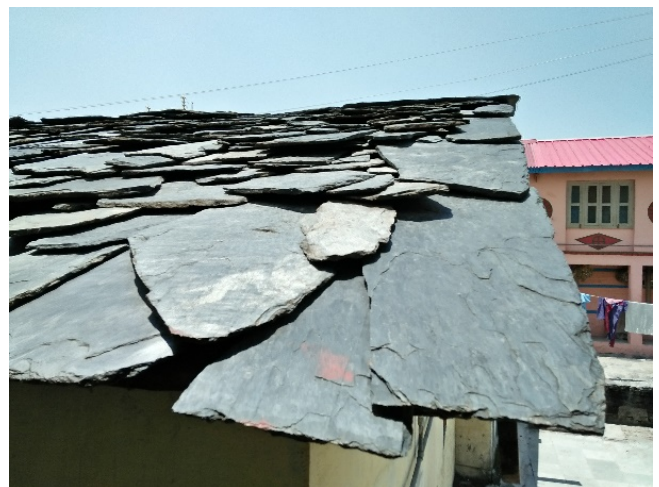
Fig. 15: Patal used as a Roof Covering
